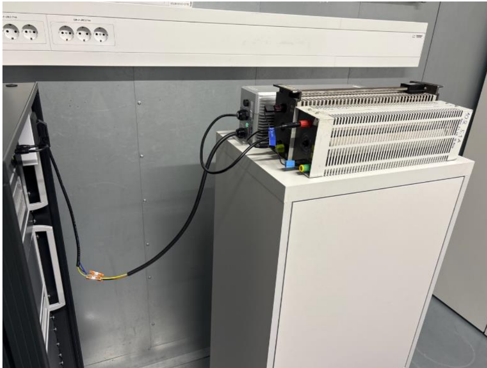
Figure 10: Voltage flicker emissions measurement
